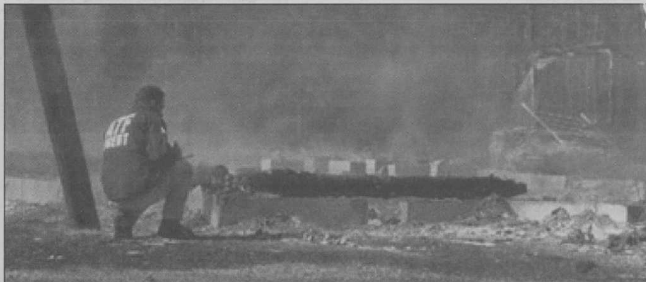
An agent from the Bureau of Alcohol, Tobacco and Firearms investigates the remains of the Morning Star Baptist Church on Tuesday near Boligee, Ala., after a fire destroyed the structure earlier that morning. Officials suspect arson.
