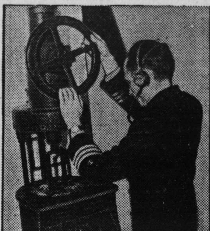
The Chart Room, testing the radio direction-finder. By noting the readings of the maximum, checked by the minimum, intensities of any two known light-houses' call letters, the position of the ship can be calculated.
