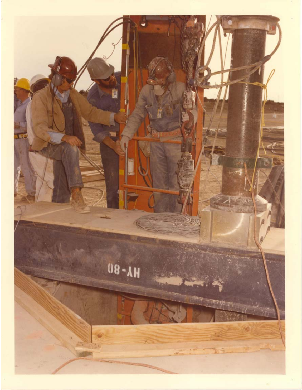
20 Mine rescue cage
