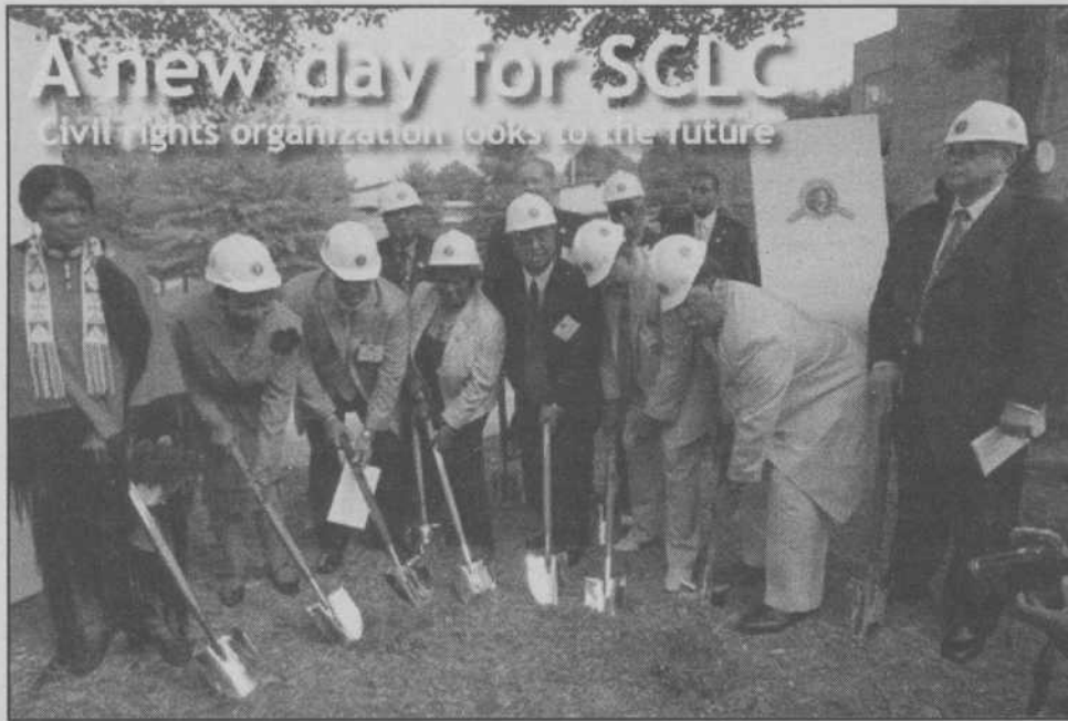
Shovels in hand and hardhats on their heads, various dignitaries gather for the groundbreaking of the Southern Christian Leadership Conference's new headquarters.
