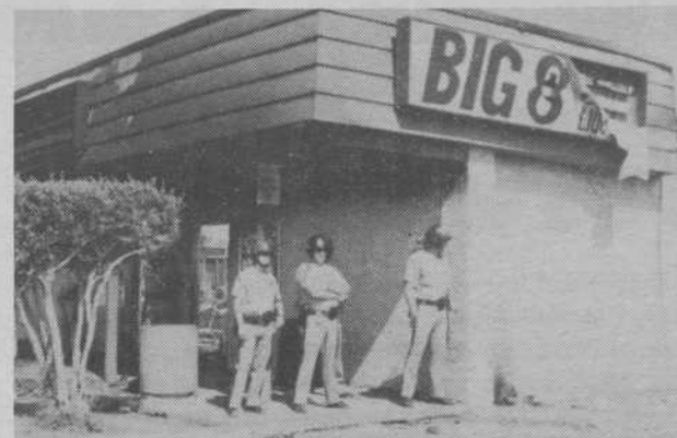
Criticized for not coming to the rescue of the Nucleus Plaza complex during the night, the police stand guard over a empty shell of a building. Photos by Savoy/LVS-Voice
