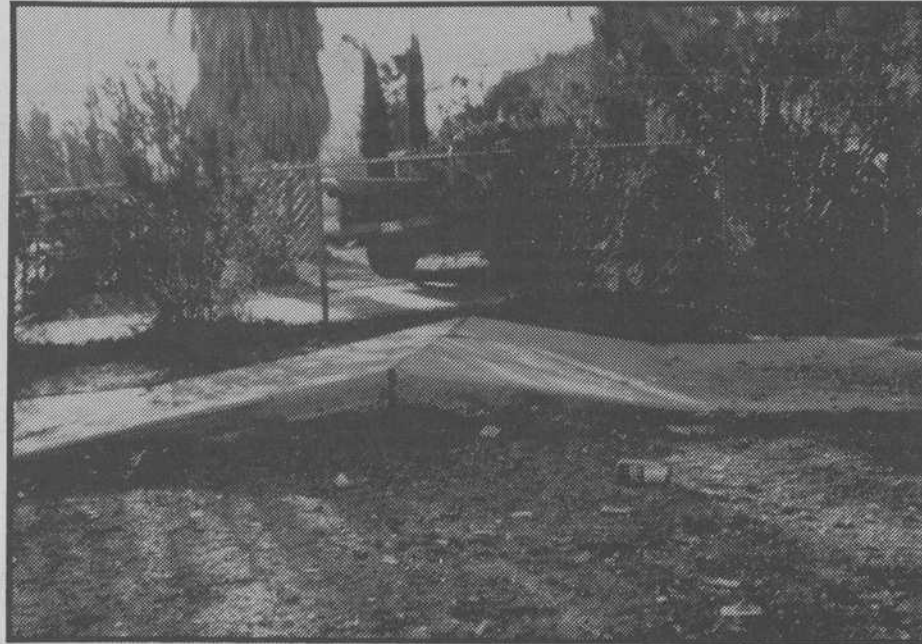
SCENES FROM WINDSOR PARK...A buckling sidewalk...
