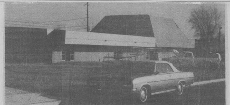
PICTURED ABOVE is the Community Baptist Church, Henderson, currently under construction and pastored by Rev. Sam Roberson. The $150,000 structure is located at 245 Foster Ave. and sits on an acre of land opposite the City Recreation Park surrounded by a beautiful setting of modern homes and apartments. It is anticipated that the church will officially open
