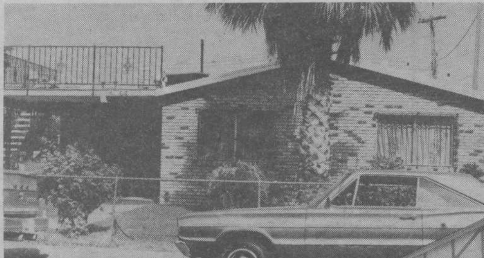
Exterior remodeled — Installed used brick veneer carport and sundeck (Regal Estates)
