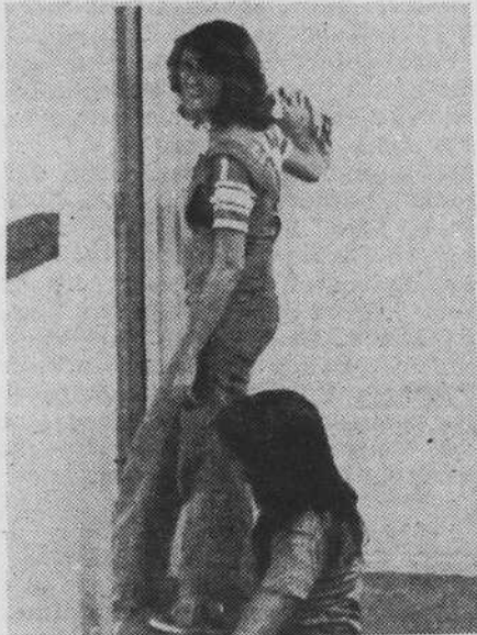
Carolyn Cantrell and Sarah Schirmer look exhausted but satisfied as they near completion of the project of painting the Easter Seal Building.
