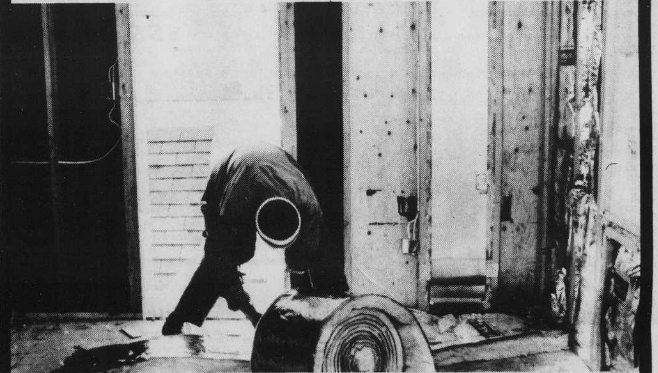
Most homes built in the days when energy was plentiful and cheap do not have enough insulation—but insulation can be added to any house, even if some already exists. Here an insulation contractor is shown working on the outside walls of a new home. If wall space is accessible the type of material in the foreground can be used. This type of insulation is called blankets and comes in rolls.
