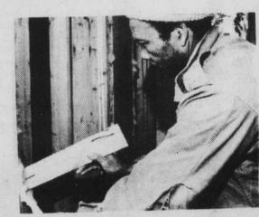
Cracks and very narrow spaces, such as those around window framing, should be stuffed by hand with loose wool (scrap). Install insulation around heating ducts and water pipes to keep them warm, particularly on outside walls.
