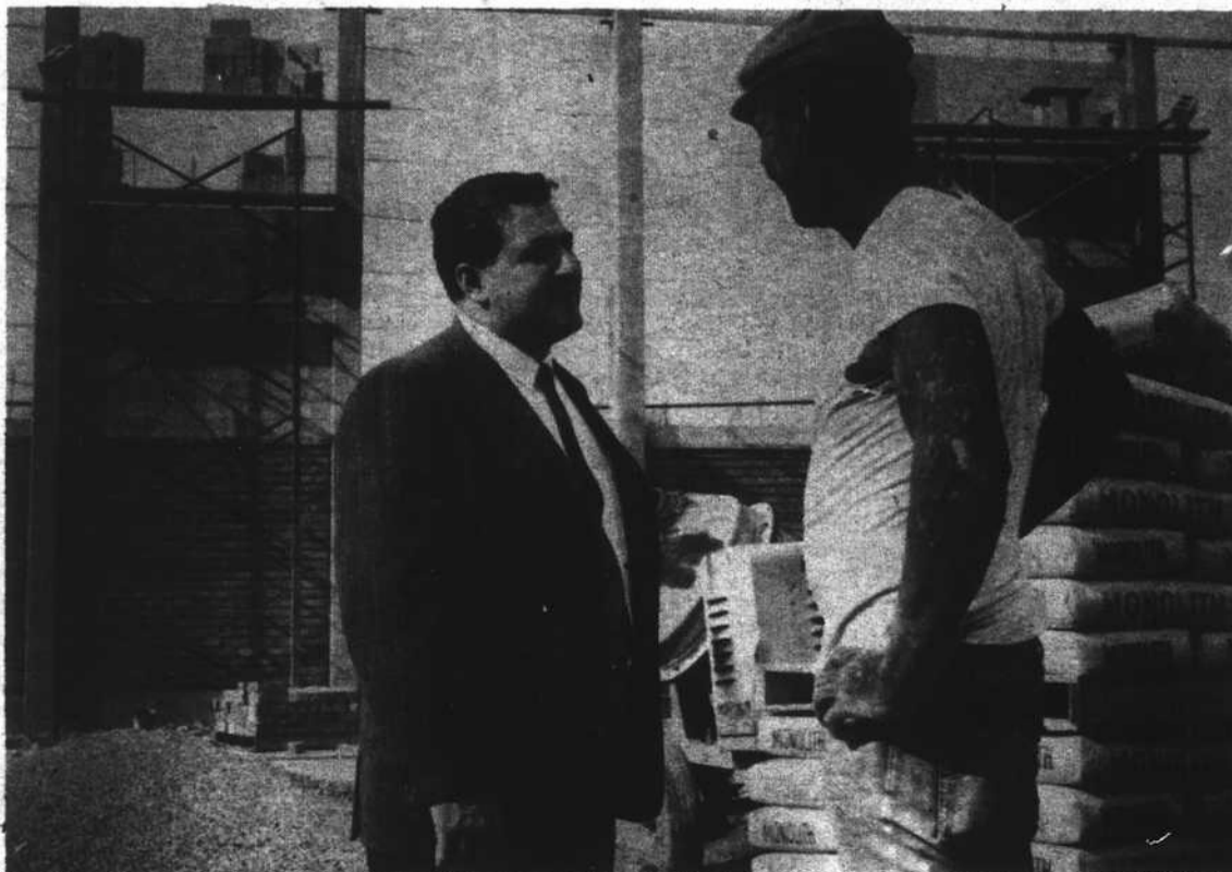
CITY COMMISSIONER PHIL MIRABELLI (left) inspects work on new gymnasium now being constructed at Doolittle Recreation complex at Lake Mead Blvd. and 'J' St., West Las Vegas
