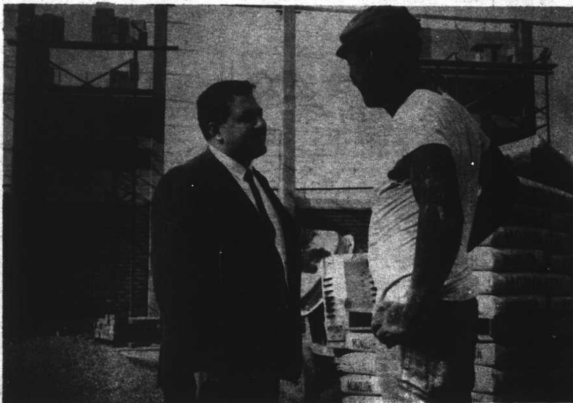
CITY COMMISSIONER PHIL MIRABELLI (left) inspects work on new gymnasium now being constructed at Doolittle Recreation complex at Lake Mead Blvd. and 'J' St., West Las Vegas
