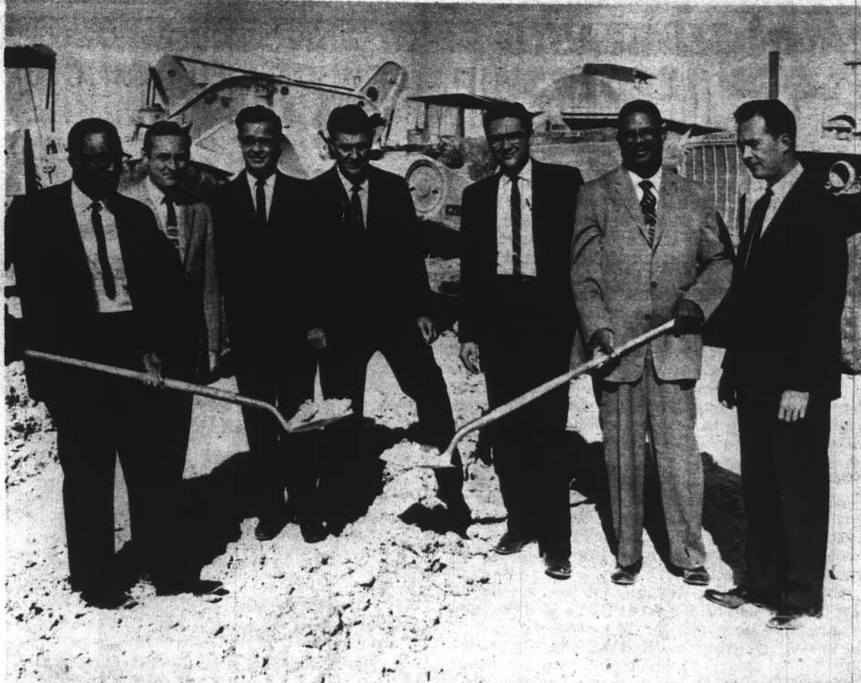
WINDSOR PARK DEVELOPMENT LAUNCHED —One of Southern Nevada's most ambitious housing projects is now officially under way following groundbreaking ceremonies at Windsor Park in North Las Vegas. Participating were (from left) Rev. Prentiss S. Walker, Greater Faith Baptist Church pastor; Ben Kemperman, sales manager, Southwest Gas Corp.; Leo Anderson, FHA service supervisor; A. B. (Duke) Ellington, vice president and general manager, Windsor Park Enterprises; Boyd Bulloch, North Las Vegas Mayor pro tem; Bishop C. C. Cox, Upper Room Church of God in Christ pastor, and William Sharpe, assistant cashier, First National Bank of Nevada. Development will consist of 476 moderately priced single family homes, 275-space mobile home park and sites for schools, churches and commercial complexes. Initial unit of 73 three and four bedroom, two-bath homes priced at 14,700 now under construction is already more than half sold according to the developer. Subsequent units are now in the planning stage according to a spokesman for Rohr Aircraft Corporation's architectural and home-building division.
