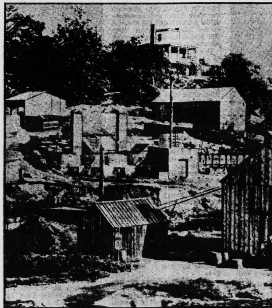
NEW refinery is on the site where John D. Rockefeller built this early Standard Oil plant about 75 years ago.
