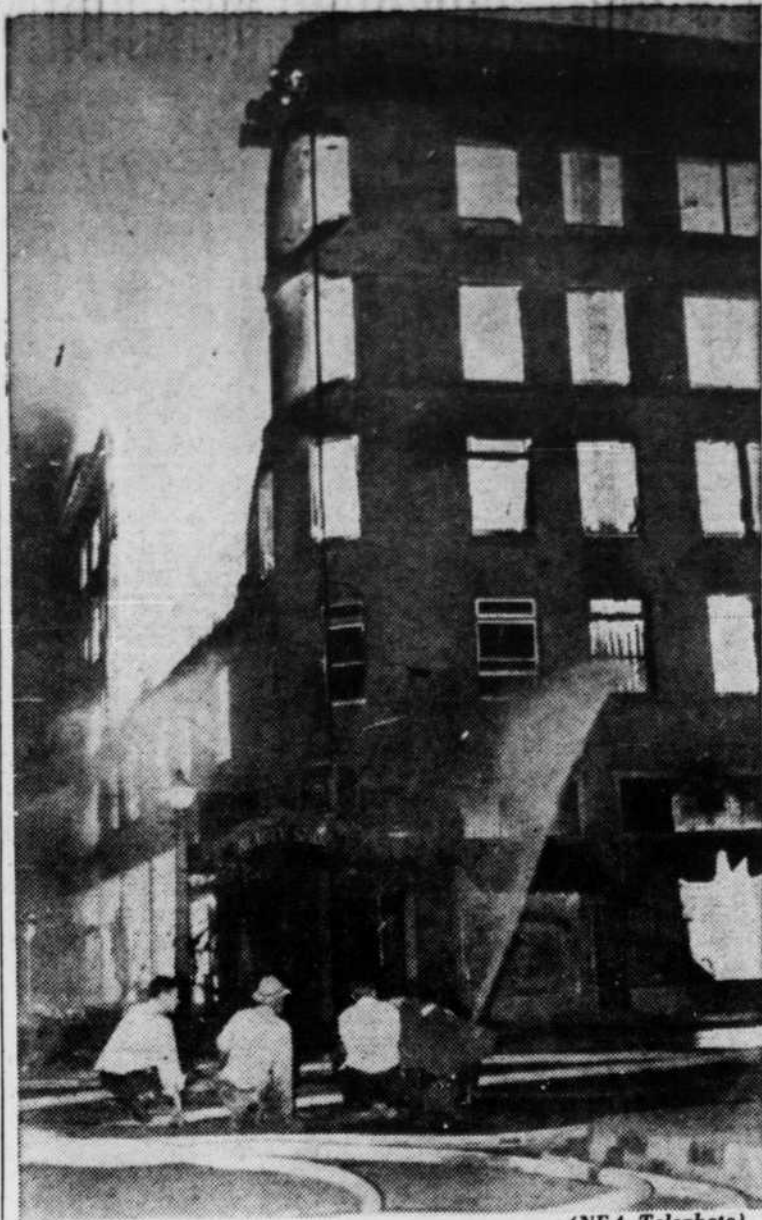
(NEA Telephoto) Flames lick gutted interior of this Modesto, Calif., hotel in fire which burned five hours and started other blazes throughout the city. One person was killed in the blaze, damage was estimated at $400,000.
