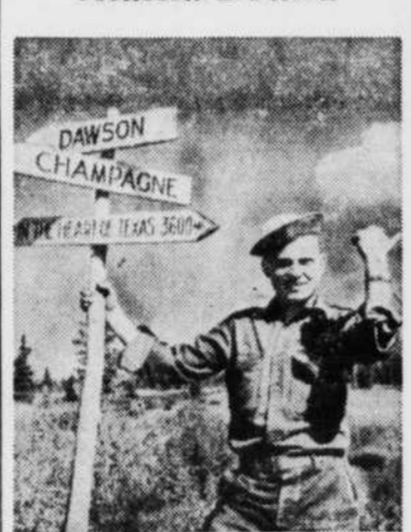
Somewhere in the middle of Canada this U. S. Army private is working on the U. S.-Canada-Alaska highway which, when completed, will play an important part in the United Nations war effort. The new highway is expected to be open by December 1.
