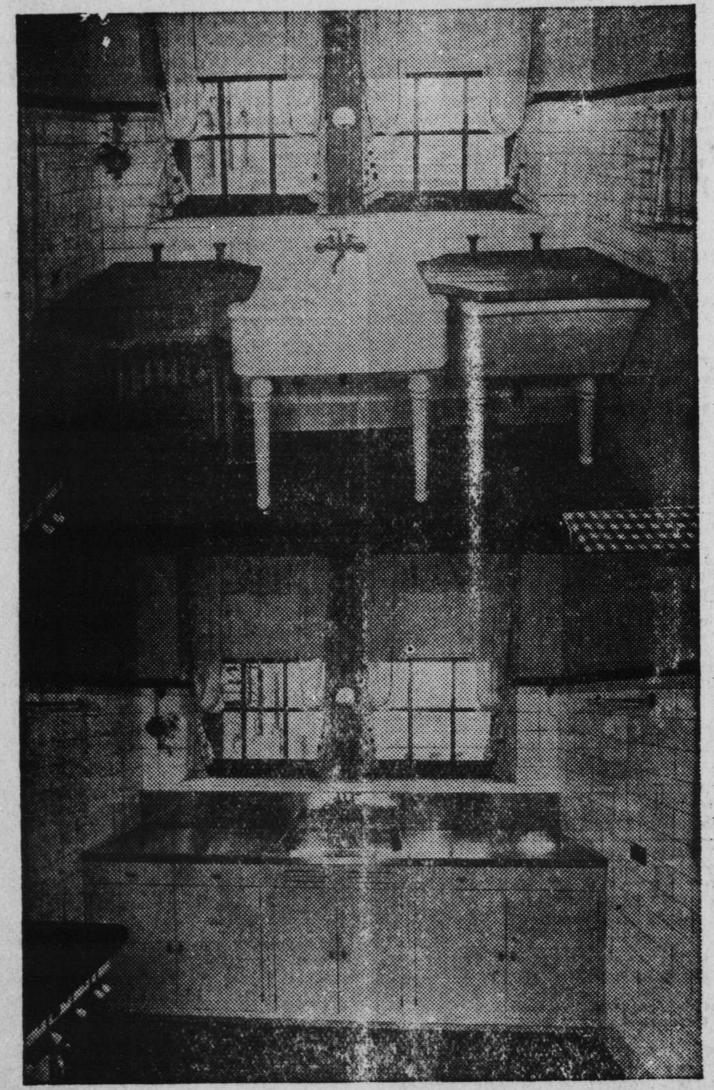
The kitchen shown above appears, at first glance, to have undergone extensive alteration and modernization. From the standpoint of working efficiency it has, but to bring this about it has only been necessary to supplant the sink, tub, and wooden drainboards with a single built-in sink and cabinet unit...
