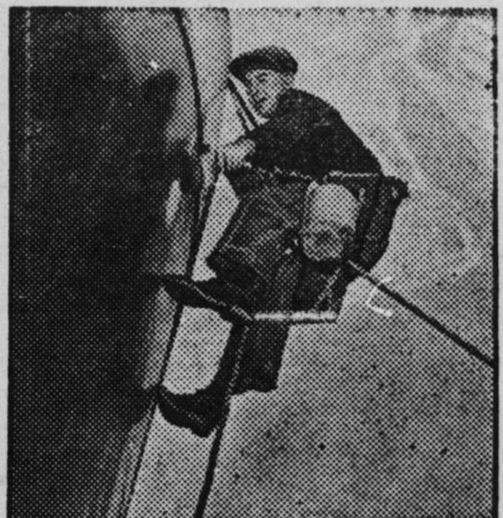
High above, in a bo's'n's chair a member of the shore gang paints the forward funnel of the ship with the Grace Line colors, green base, white band, and black top.
