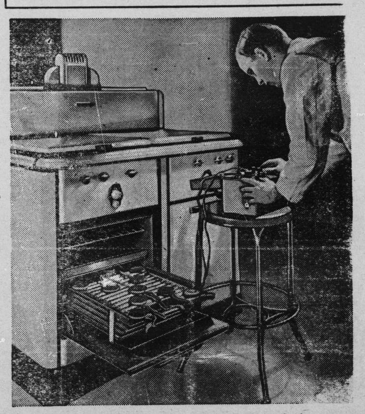
TAVE you ever wondered what a scientist looks like? Above is the II pictured conducting a broiling temperature test on a new model go range in the famous testing laboratory of the gas industry at Cleveland, Ohio. This is but one of more than 500 scientific tests a range must undergo before winning the laboratory seal of approval, which means the range will give long and distinguished service as the peer among cooking appliances.
