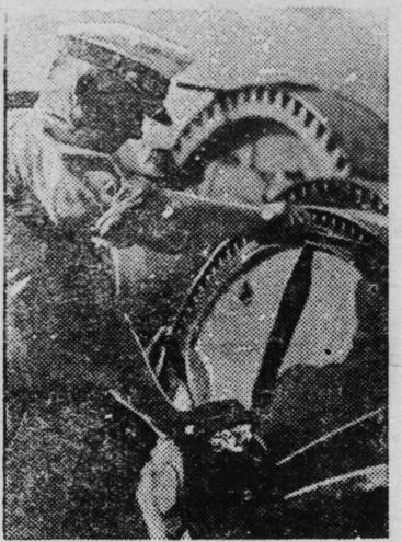
HIPS in port are beehives of industry Repairs are made: stores eplenished: cargo unloaded and caded. Derrick winches work twen r-four hours a day. As the "Santa ucia" nears New York, the ship's rpenter greases the winches o · luxurious Grace Line ship.
