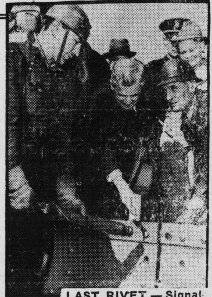
LAST RIVET — Signaling the last bit of construction work on the Golden Gate Bridge, San Francisco, the last rivet, made of gold, placed by Chief Engineer Joseph B. Strauss was driven by the crew that drove the first rivet or the job.
