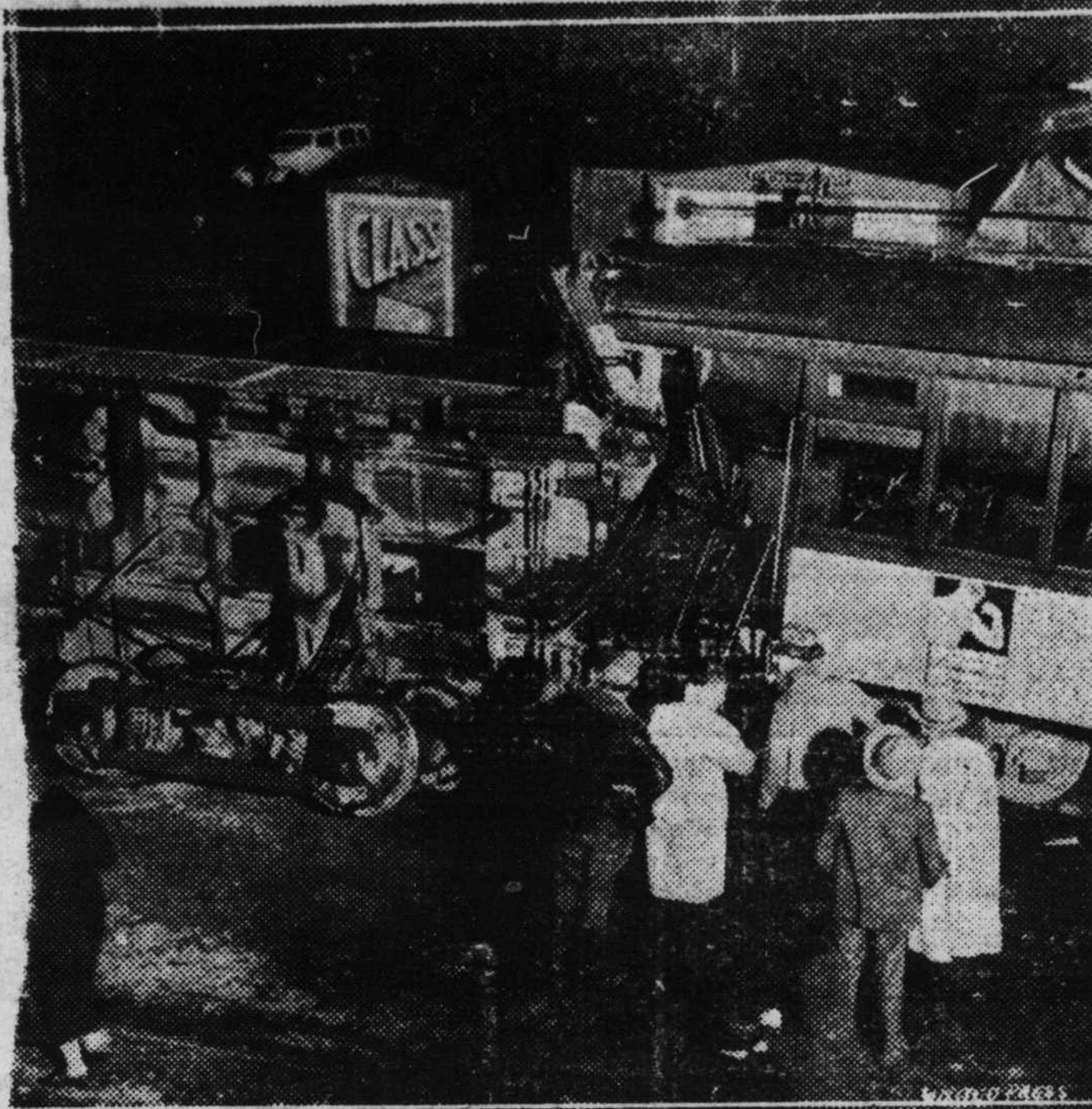
Thirteen people were injured, one perhaps fatally, when these two streetcars crashed in strike-torn Los Angeles. Investigators reported that the cars met head-on, one being turned over by the crash. It was disclosed that the wreck had been caused by a plugged switch.
