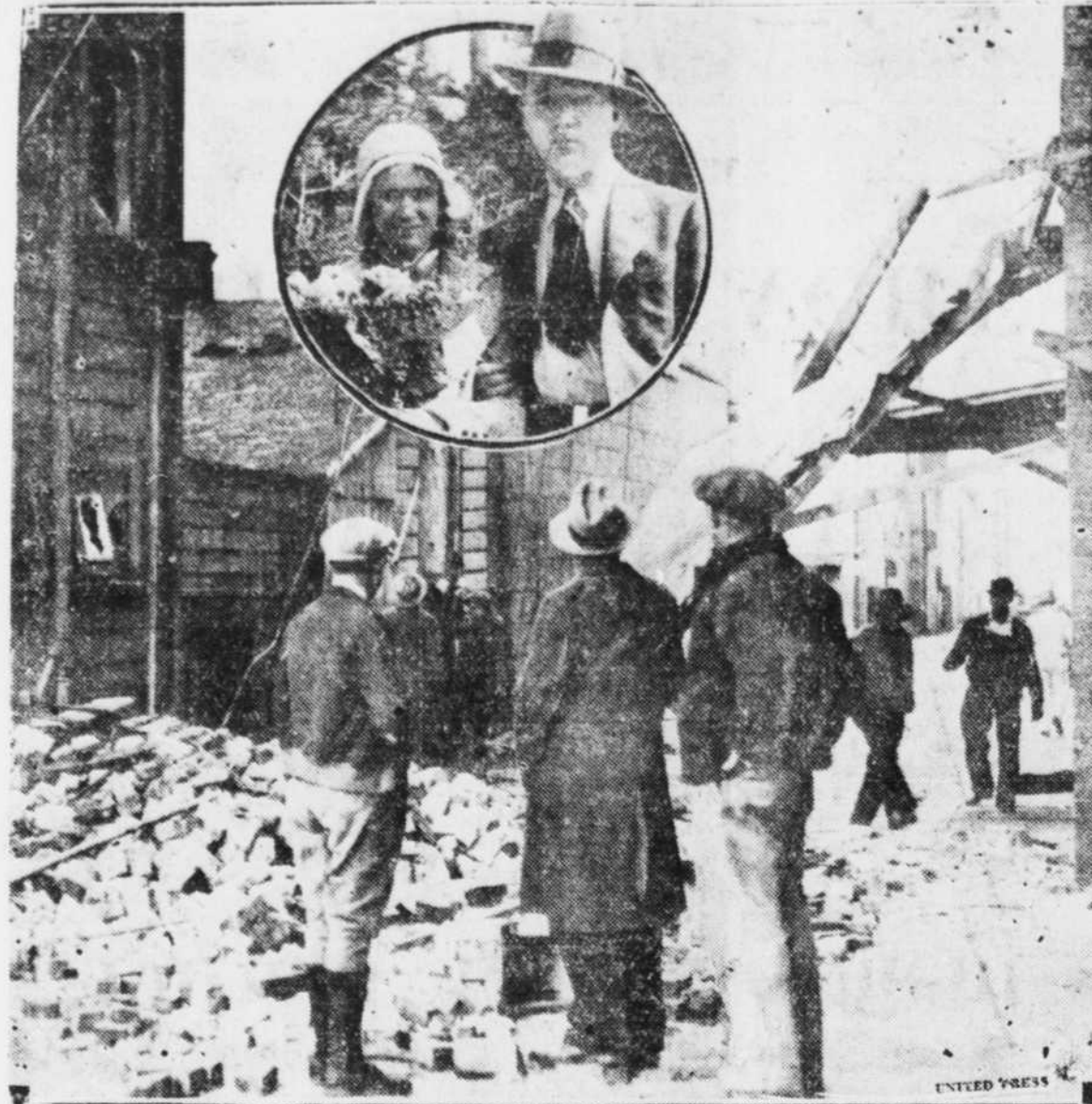
One of the most severe earthquakes California had felt in many years appeared to center at Eureka, 300 miles north of San Francisco, on the coast. There Mrs. McCutcheon, 25, was killed when a brick chimney crashed through a roof, and her husband incurred some broken bones. The above scene shows debris shaken down by the tremor. Mrs. McCutcheon and her husband appear in the inset. The quake was felt for 250 miles along the coast, and extended as far inland as Yreka, Calif., and Roseburg, Ore.
