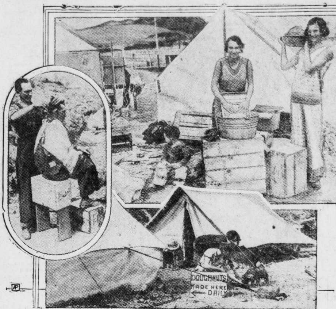
Thousands of job-squatters near the site of Hoover dam are making the best of things in their make-shift homes. Upper right shows Billie Wagner (at tub), formerly of Cleveland, and Thelma Griffin, formerly of Spokane, doing the washing. An amateur barber (left) has found a customer, and the wife of one job-seeker se's doughnuts (below) while her husband waits for work.
