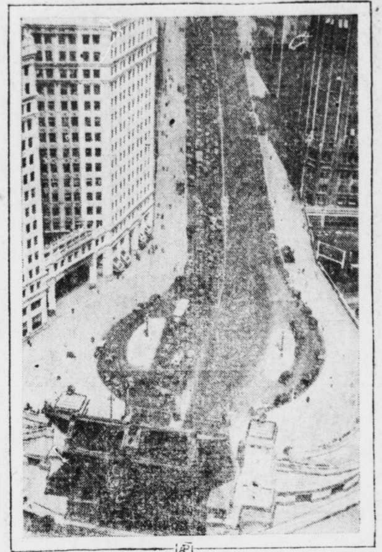
The new outer drive bridge in Chicago is expected to take about 50,000 cars a day off Michigan avenue. Above is shown "stalled" traffic on Michigan with Chicago river bridge open.
