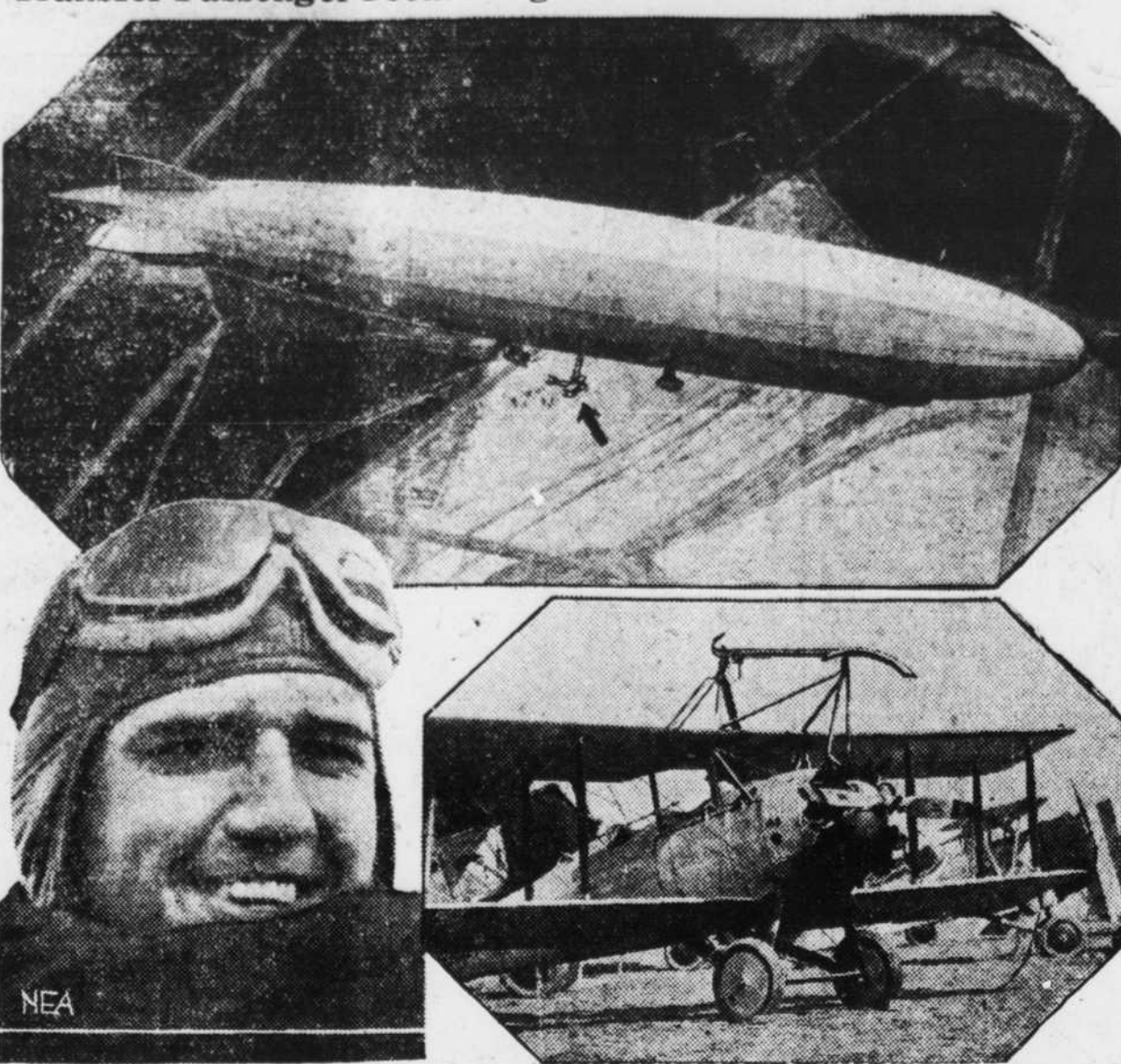
Here's how an airplane was hooked on to a giant dirigible and a passenger transferred to the plane in mid-air in the first test of the kind ever made, witnessed by 100,000 awed spectators at the National Air Races at Cleveland. Lieut. A. W. Gordon, navy flyer, below, hooked his standard navy fighting plane (shown below) to a device lowered from the Los Angeles and Lieutenants Calvin Bolster climbed down to the plane. Above is the Los Angeles over the airport, with an arrow indicating a sketch showing how the hook-up between plane and dirigible was made. The thrilling mid-air stunt was performed to demonstrate the ability of dirigibles as airplane carriers, as the two new dirigibles now being built for the navy will each carry several planes to take off and return in mid-air.
