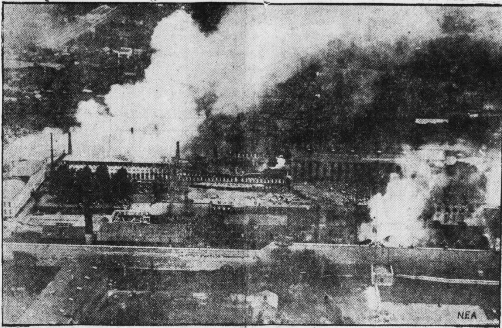
Burning of the Auburn, N. Y. prison in the spectacular mutiny of 1700 convicts, who set fire to a half-dozen buildings in a sensational break for freedom, is strikingly portrayed in this exclusive Las Vegas Age's NEA Service aerial photo. Firemen are shown on the high pentagonal walls, vainly fighting the blaze, while guards inside the prison quadrangle bat (red inmates who had armed themselves with guns and ammunition from the prison arsenal. Fire destroyed the furniture plant, the canteen shop, the prison kitchen, the machine shop, the State shop and the finger-printing office, with its Bertillon records. Two convicts were killed and more than twenty men wounded in the fighting. Four prisoners escaped.
