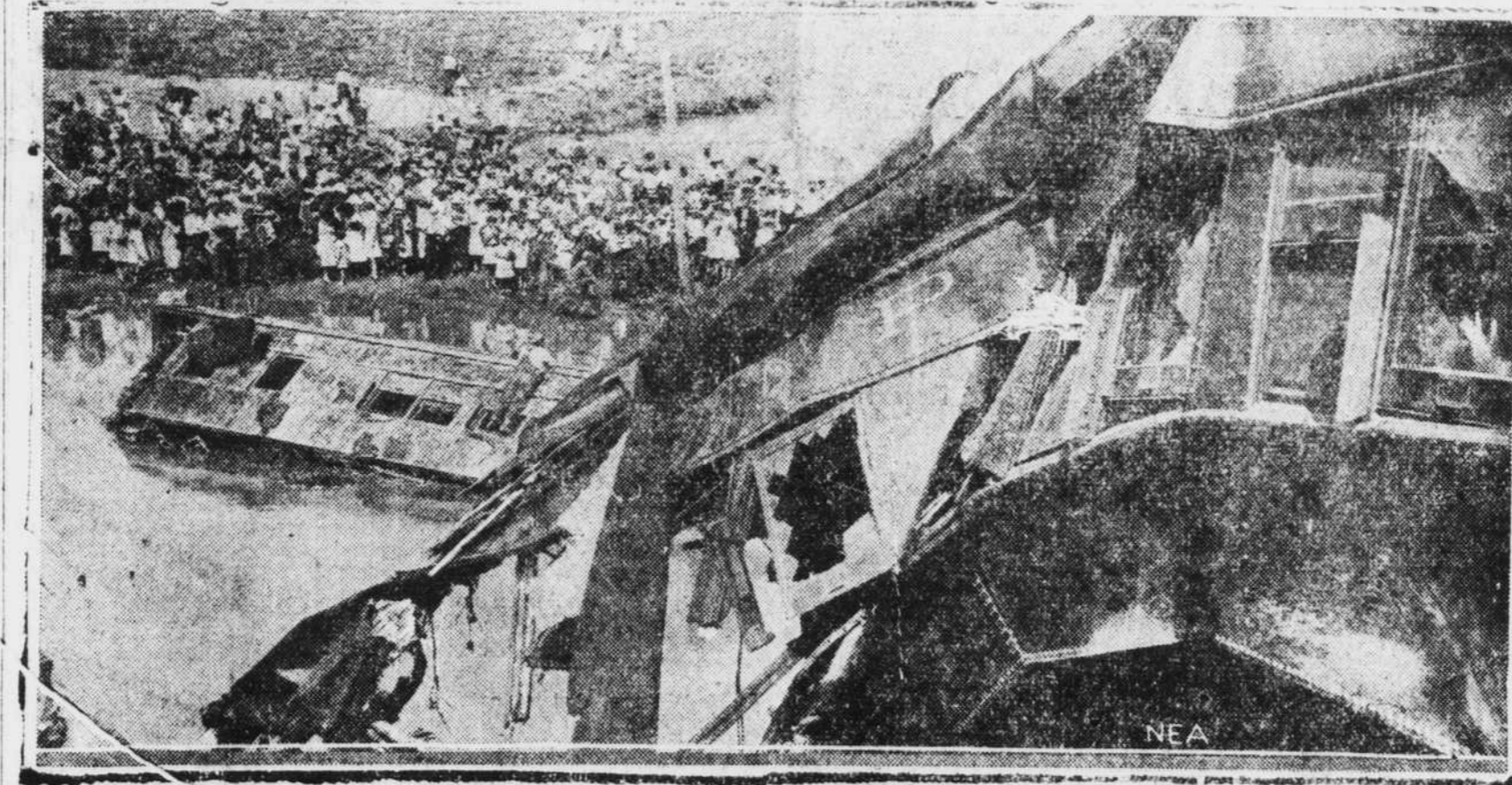
Here are some of the scenes near Stratton, Colo., Thursday when the crack Eastern Express of the Rock Island Railway crashed through a weakened bridge carrying several coaches and their sleeping occupants into the torrential creek, with death for nine, and injury for others. Photos show various views of the havoc, including a glimpse directly across the creek, with the bare supports showing where the rails and span were a way.
