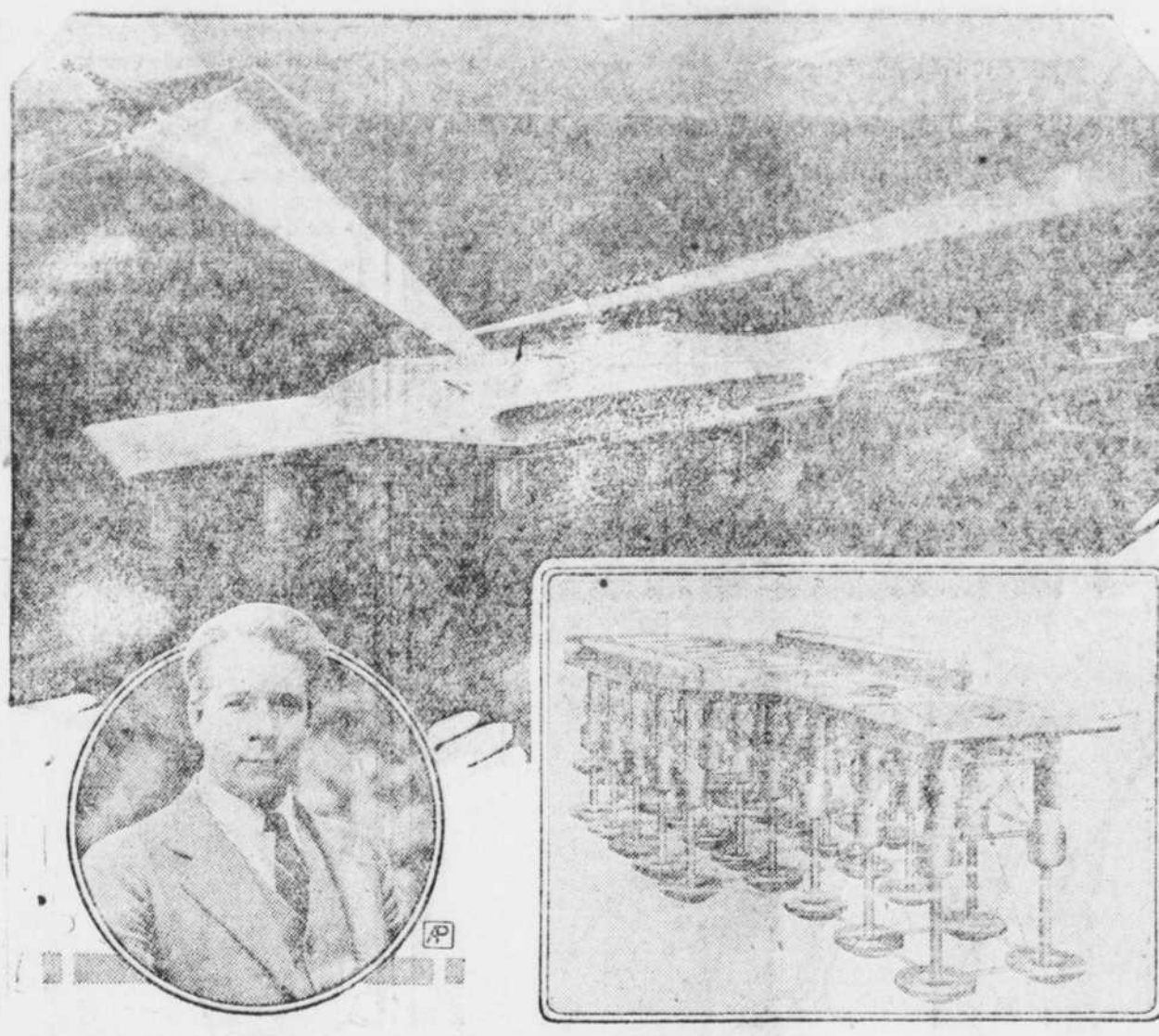
Construction of the first of a chain of "floating airports" to span the Atlantic ocean is scheduled to start in July. A striking night scene of the seadrome from the air is pictured by the artist (above), while the model (below) shows the details of its construction. The seadrome was conceived and designed by Edward R. Armstrong (inset).
