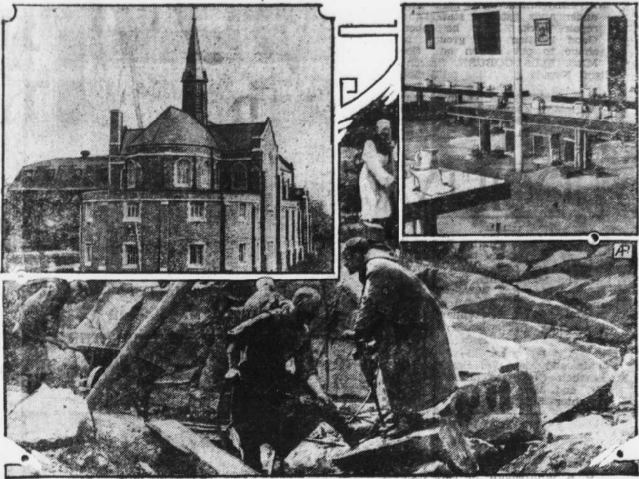
A blue-gray chapel (upper left) rising from a hill in Cumberland, R. I., is the reward of years of labor on the part of Trappist monks (below) who quarried the stone and helped erect the structure. The monks live and work under a rule of silence. Upper right is the dining room in the chapel basement.
