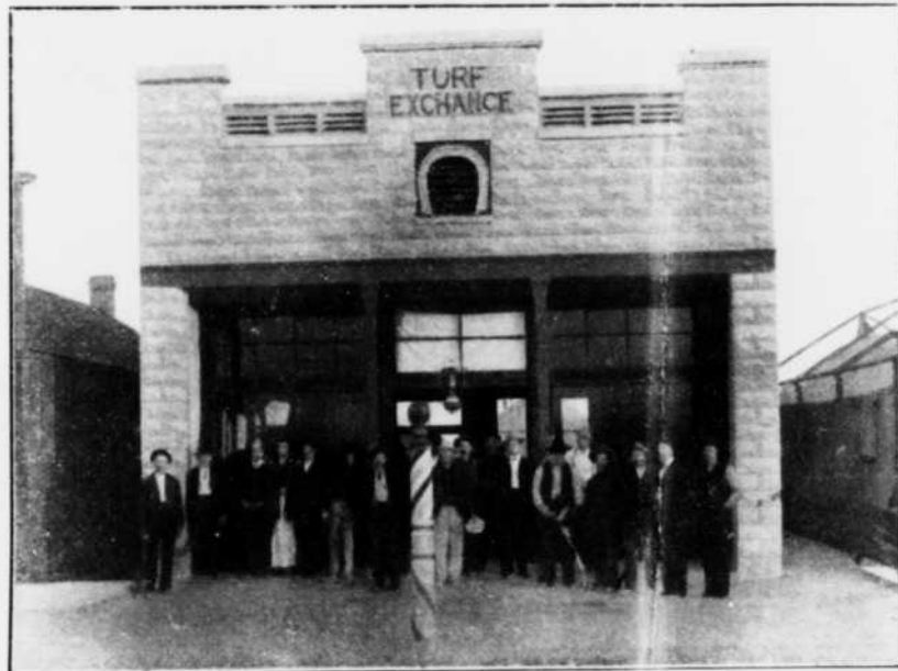
McKNIGHT & FARRELL, Proprietors A creditable saloon building on First Street, built of concrete blocks manufactured in Las Vegas
