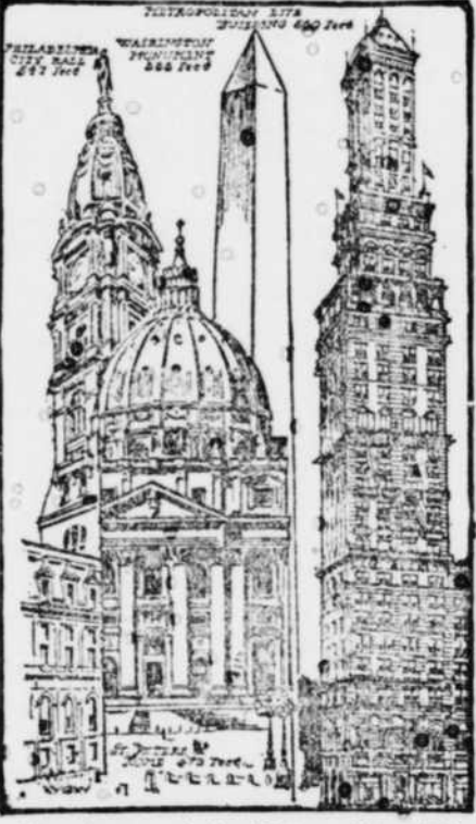
New tower of the Metropolitan Life, in New York City, to be the tallest structure in the world.
