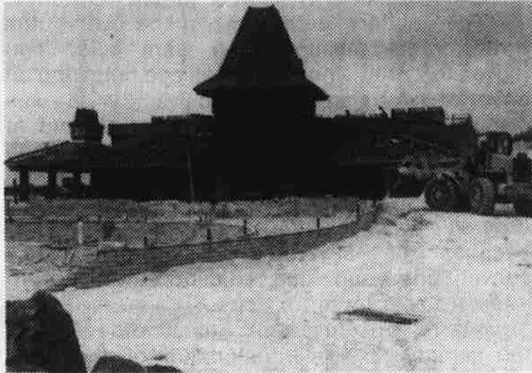
Scandia Family Fun Center in Las Vegas - under construction.
