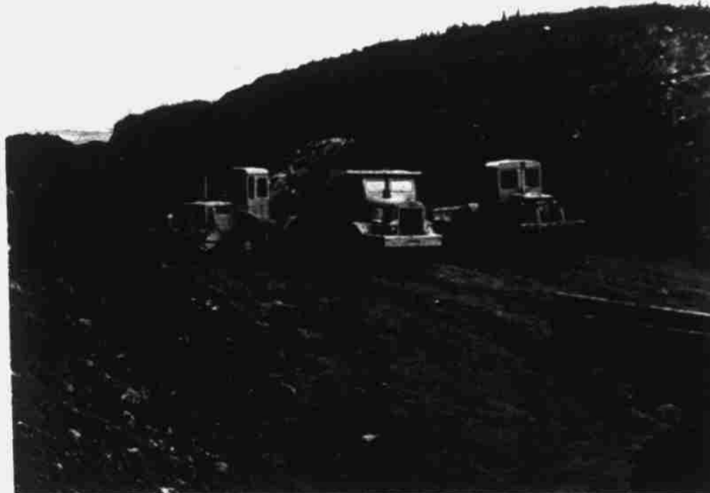
TRUCKS HACK OUT PATH FOR NEW ROAD TO KIBBITZIM IN GOLAN HEIGHTS. HERE IS EXAMPLE WHERE YOUR MONEY GOES WHEN YOU SUPPORT COMBINED JEWISH APPEAL DINNER, MAY 25 AT CAESARS PALACE. (ISRAEL SUN PHOTO)
