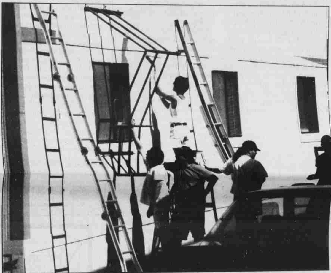
Students and faculty build Architectural art on the trailers on Brussels Road.
