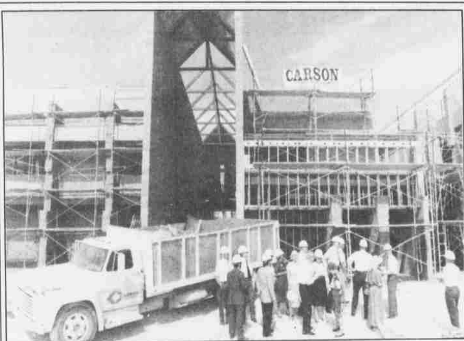
The Desert Research Institute building under construction
