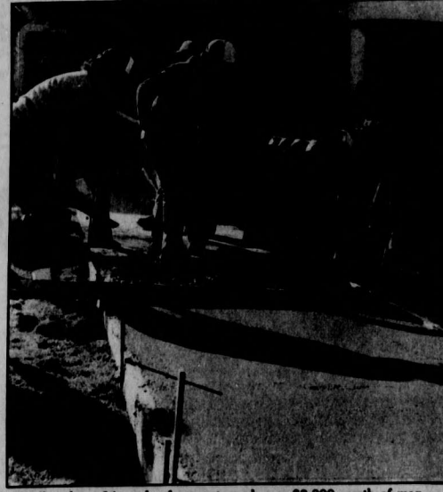
Finally, about 24 yards of concrete and over $2,000 worth of man power alleviated the problem, and students put their boots back in the closet.
