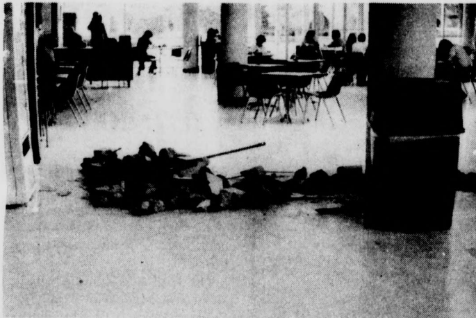
This pile of rubble marked the beginning of the Union renovation.
