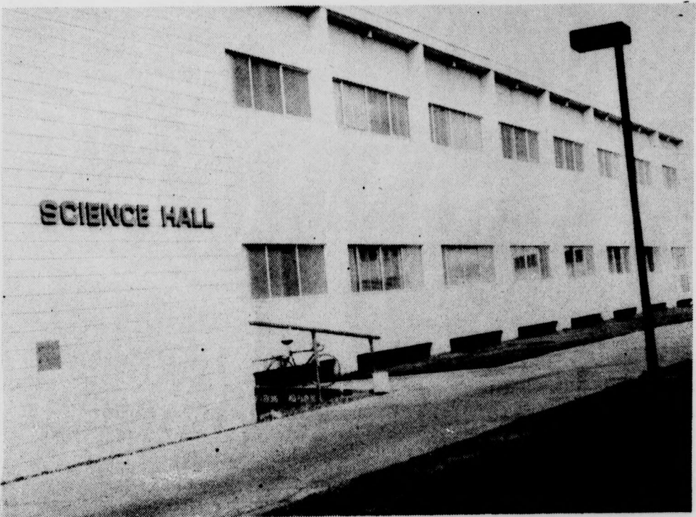
Built in 1961, the old science building has yet to be named. Once the site of all the science classes, it now houses the physical science department.
