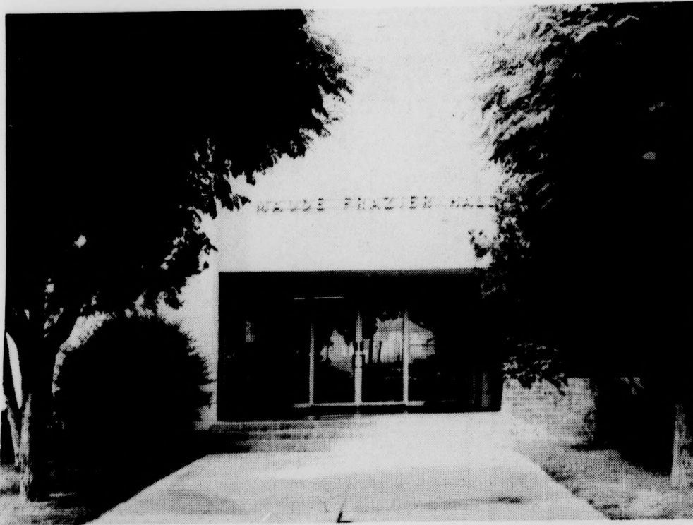
Named for Prominent Las Vegan Maude Frazier, this building once served as a 'multi-purpose' facility. It housed two classrooms, a chemistry room, a library, and a bathroom with basketballs stored in the tub.
