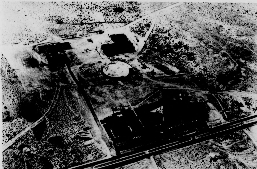
This aerial photo taken in 1963 shows the newly born Nevada Southern University campus in its early stages. The building under construction is the Library. Also shown are the Bio Labs, P.E. facilities, Grant and Frazier Halls, and a young Maryland Pkwy. The name was not changed until the late 1960's.
