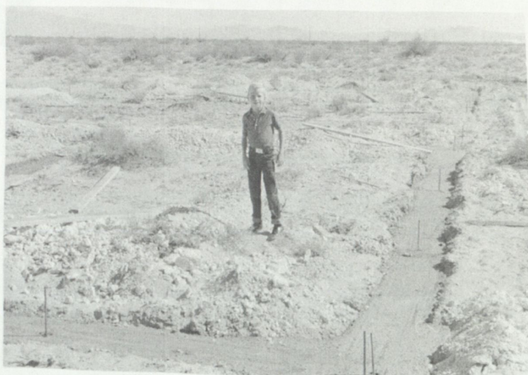
Checking the foundation. Neil Daseler
