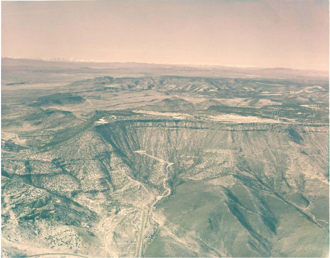
Photo 19: Circa 1968 G-tunnel access road and portal setting on Rainer Mesa.
