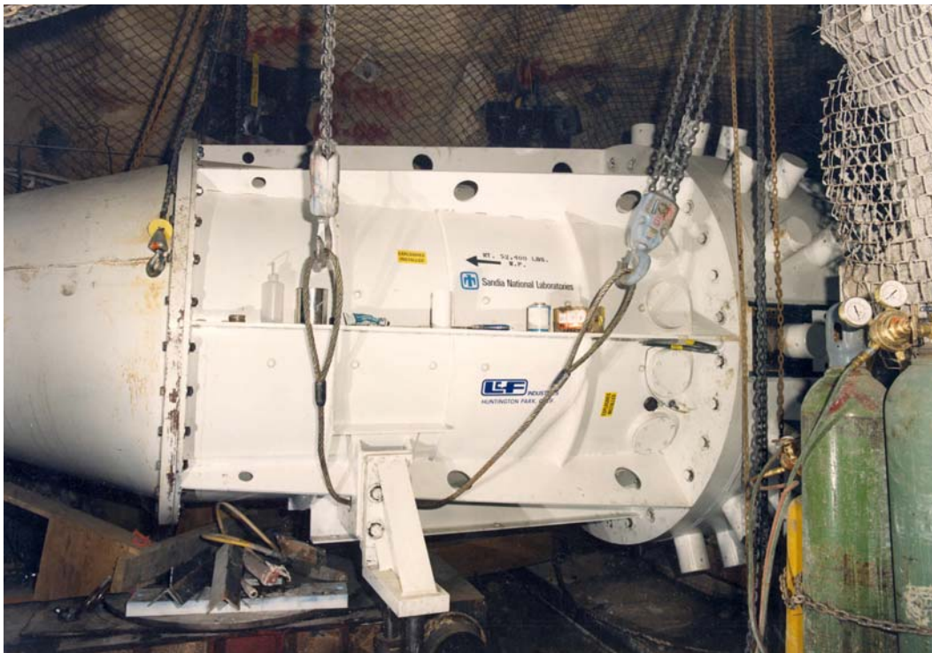
Photo 16: DIAMOND BEECH FAC mounted on LOS pipe.
