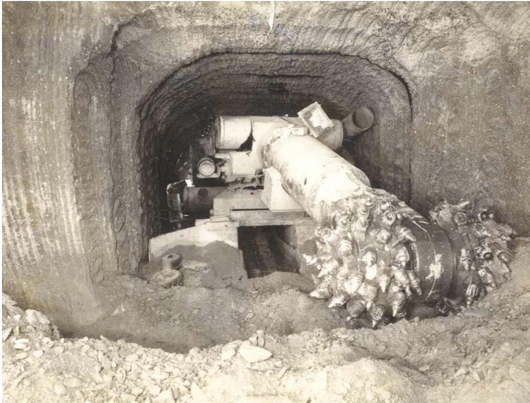
25 – Alpine Miner in N-Tunnel breaking through LOS drift
