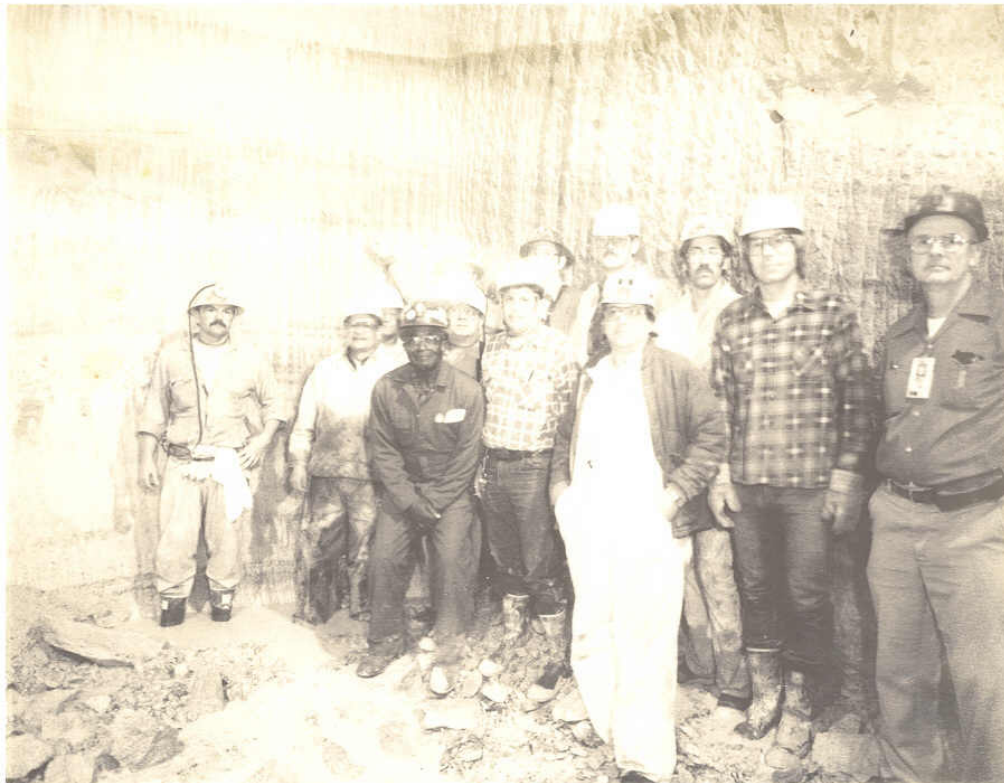
16 - Crew at U12 N-Tunnel (Bruce Wilhelm is at far right)
