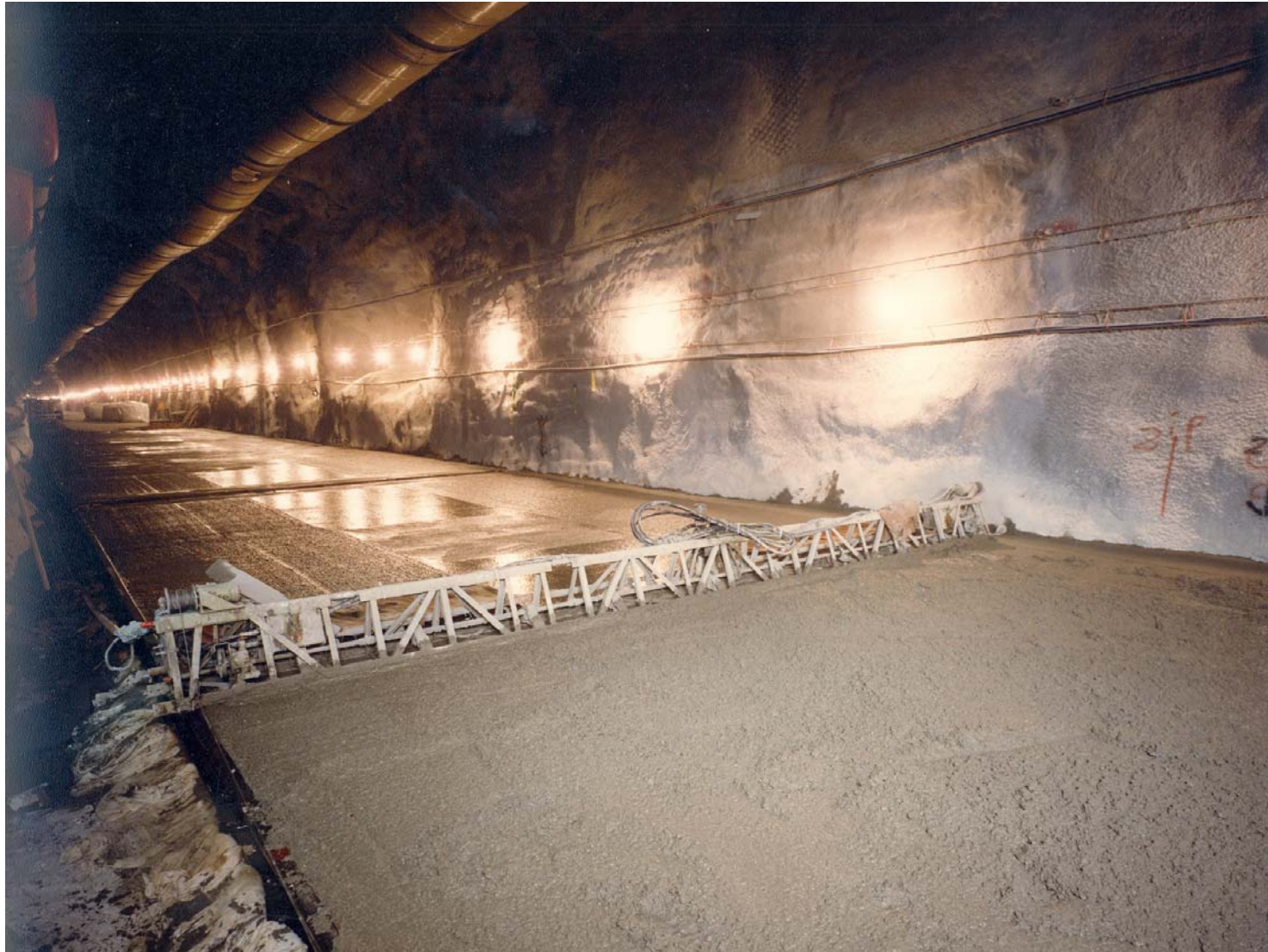
30 – Pouring concrete on the invert at P-Tunnel
