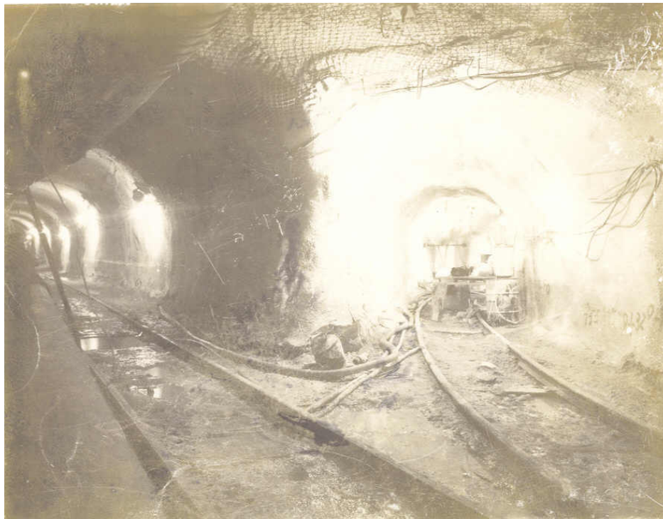
14 – N-Tunnel Area 15 at A and B drift
