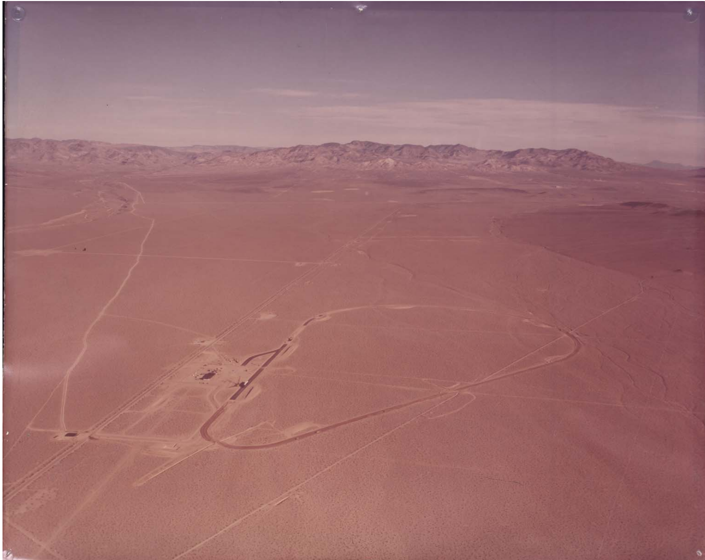
4 – Aerial Photo of Area 25 and the MX Silo and Racetrack
