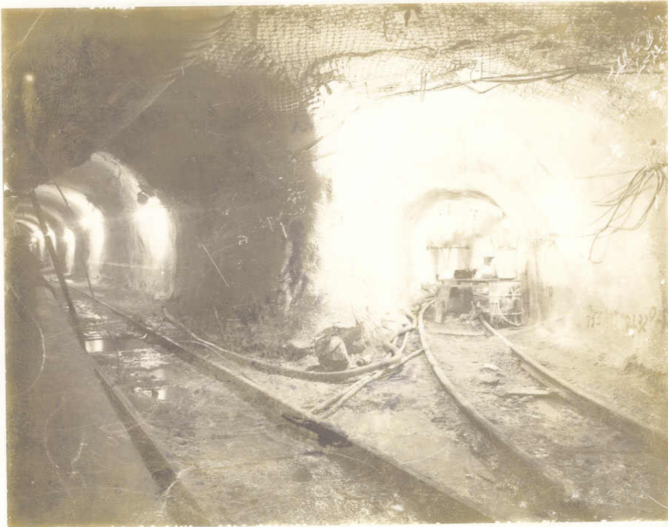
14 – N-Tunnel Area 15 at A and B drift
