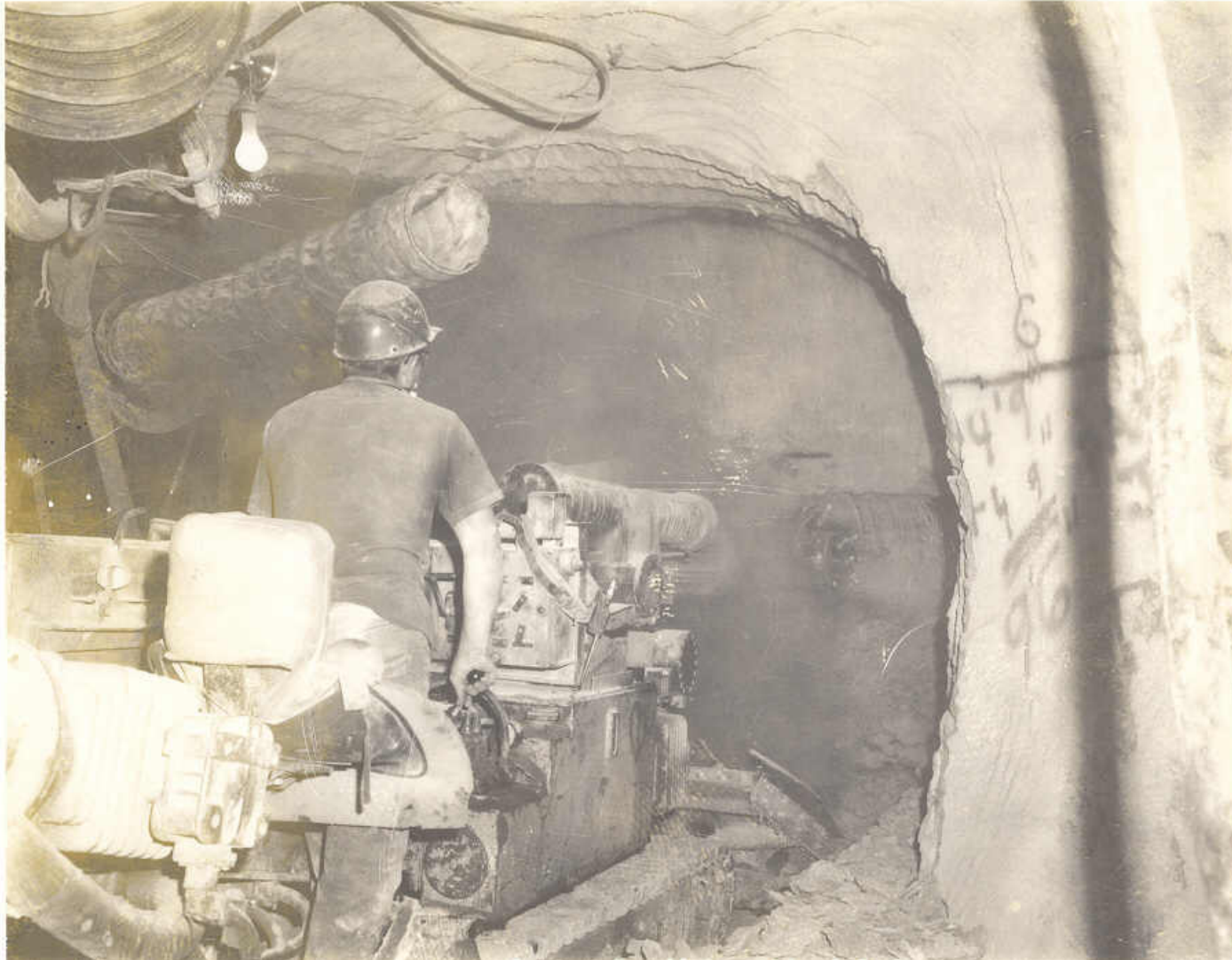
17 – Waid Tadlock operating an Alpine Miner in N-Tunnel
