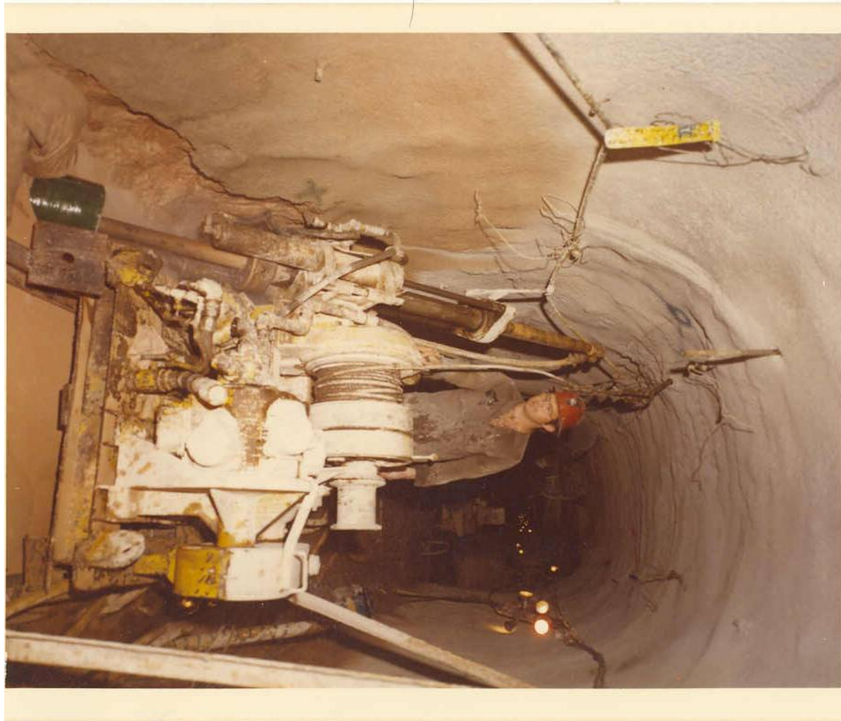
12 – John F. Campbell next to a Diamond Drill Rig in U12N Tunnel
