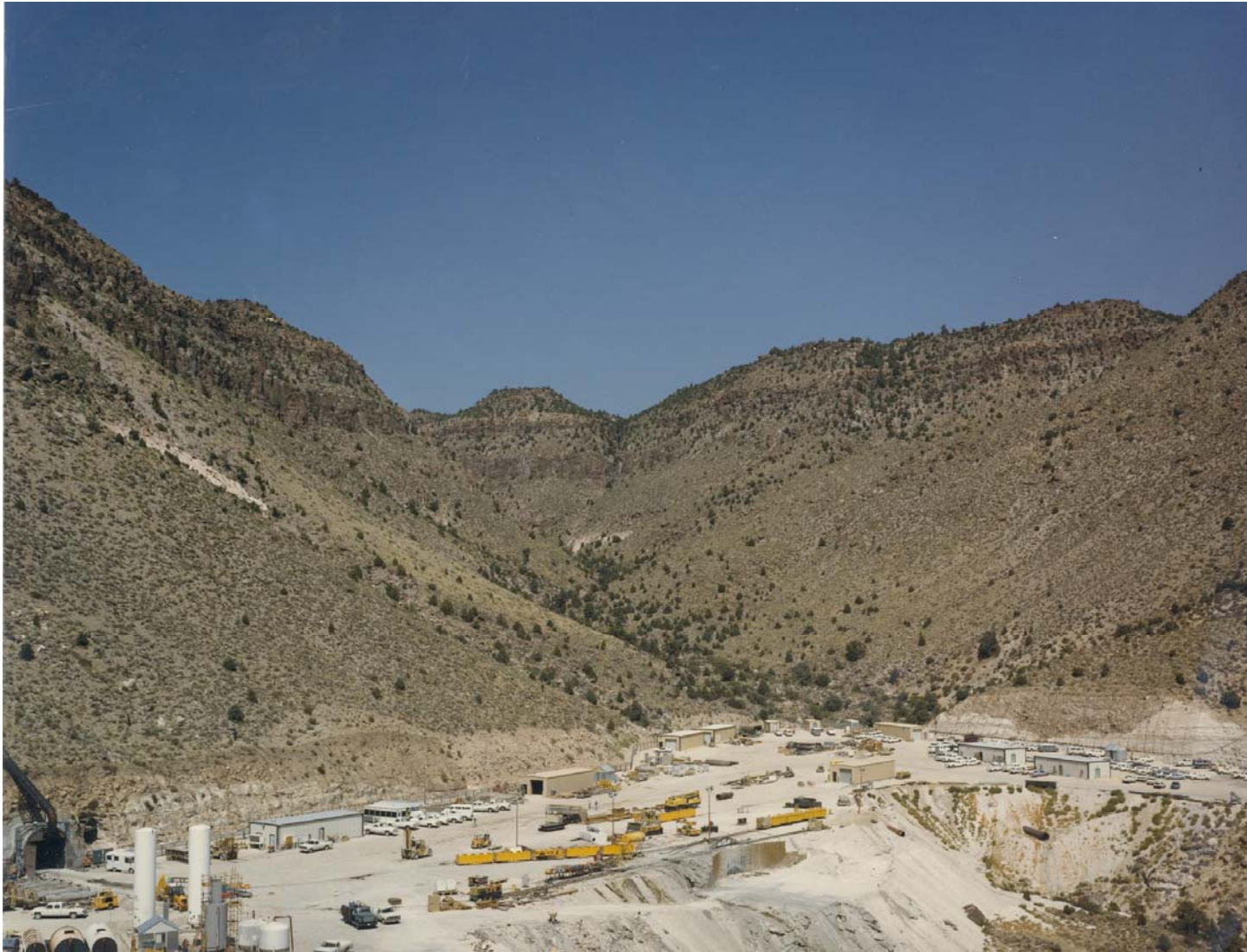
29 – P-Tunnel Portal and Yard
