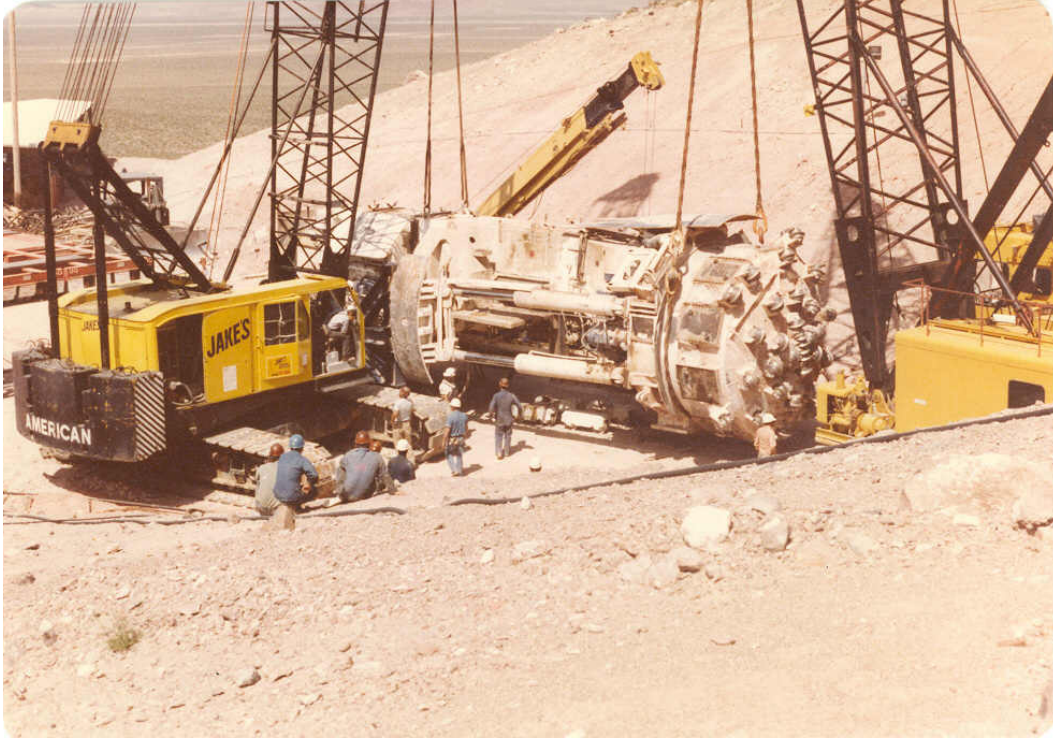
15 – Two-crane pick up of a Tunnel Boring Machine
