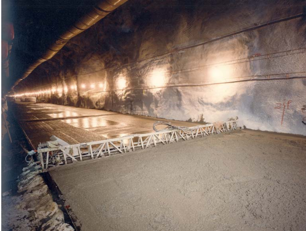
30 – Pouring concrete on the invert at P-Tunnel
