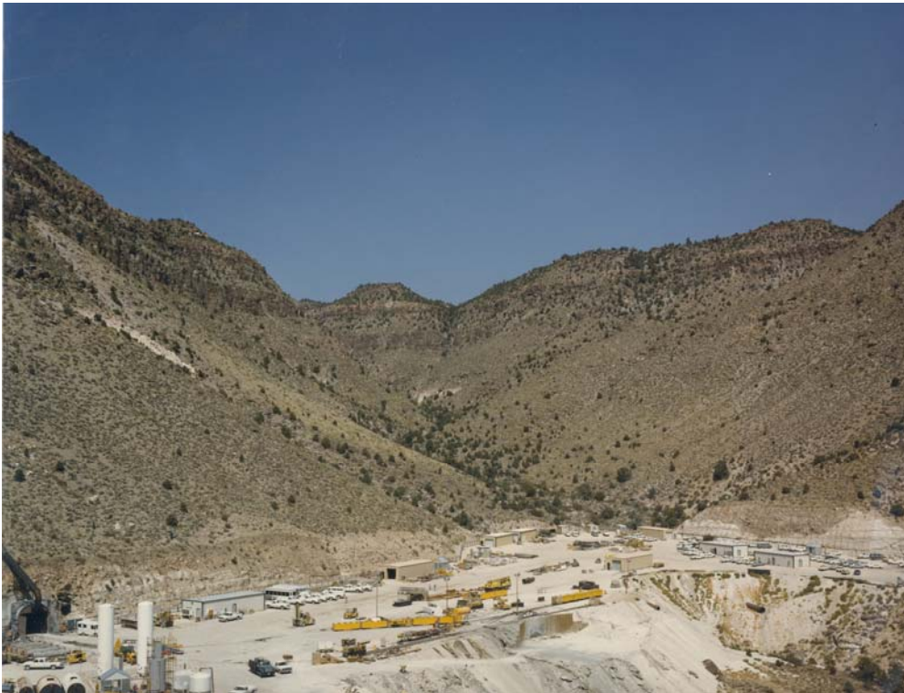
29 – P-Tunnel Portal and Yard
